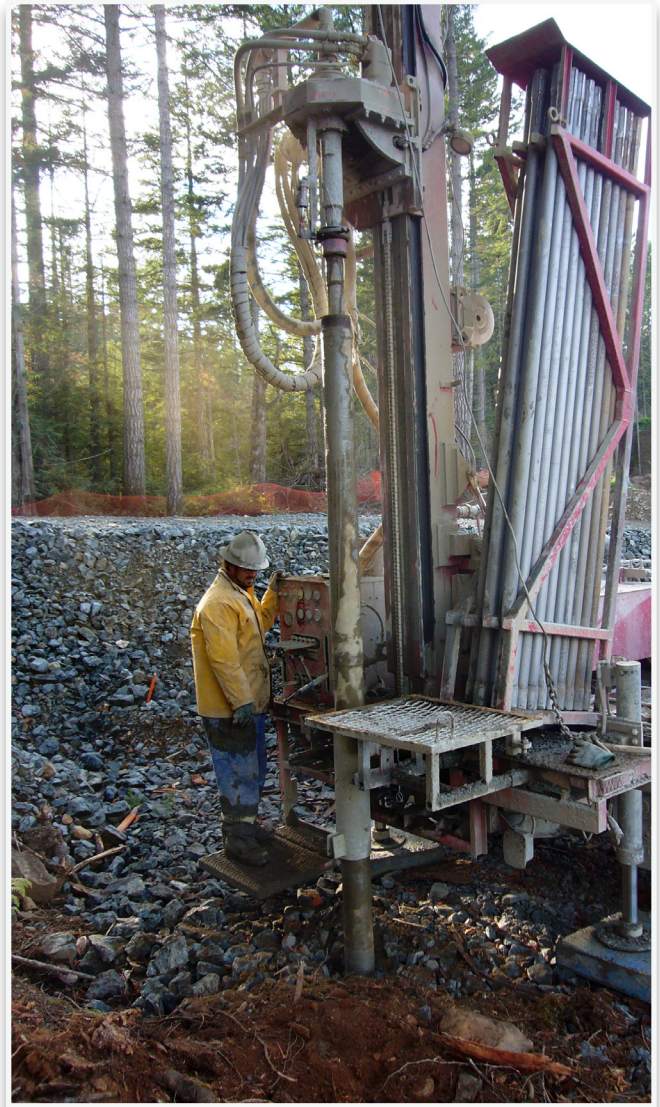
Closed-loop vertical GHX air rotary drilling
