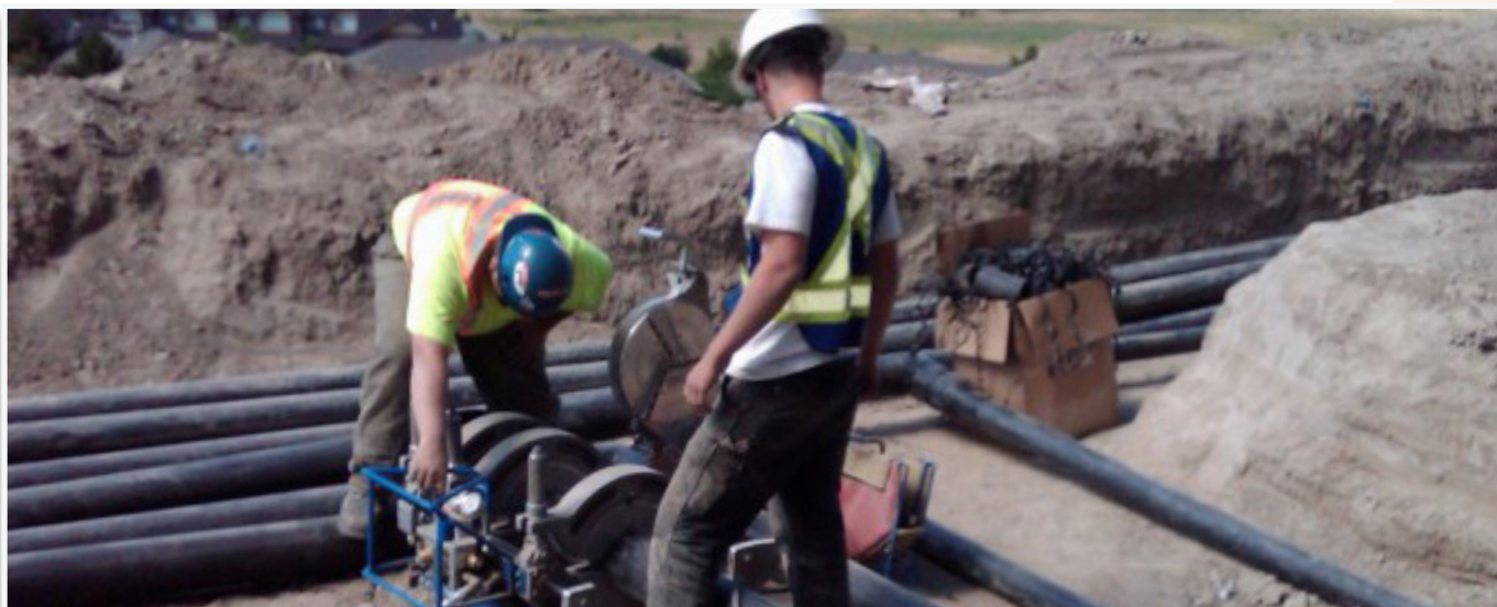
Large diameter pipe fusing
