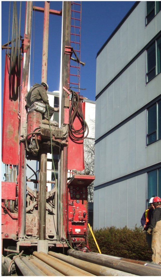
Open-loop Groundwater GHX Well Installation
