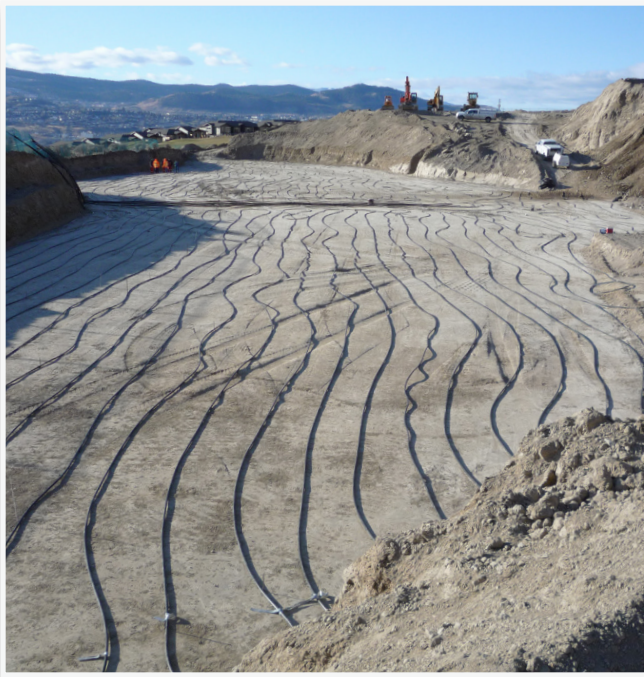
Horizontal closed loop ground heat exchanger
