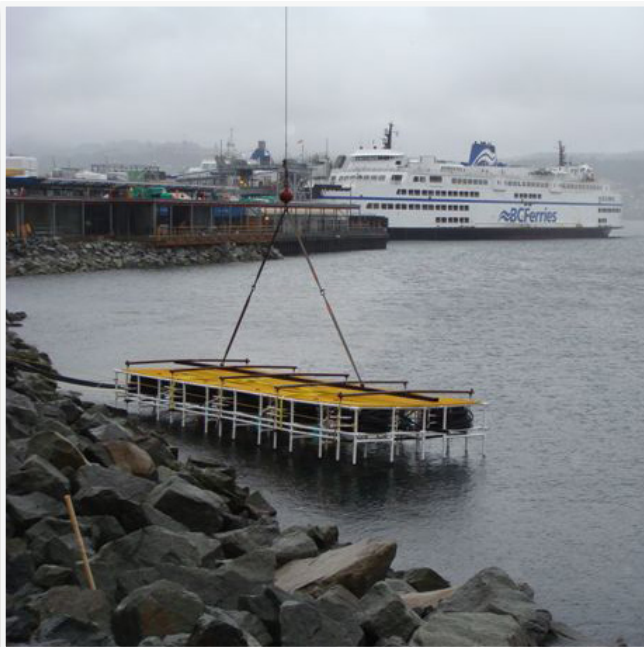
Closed loop surface water heat exchanger
