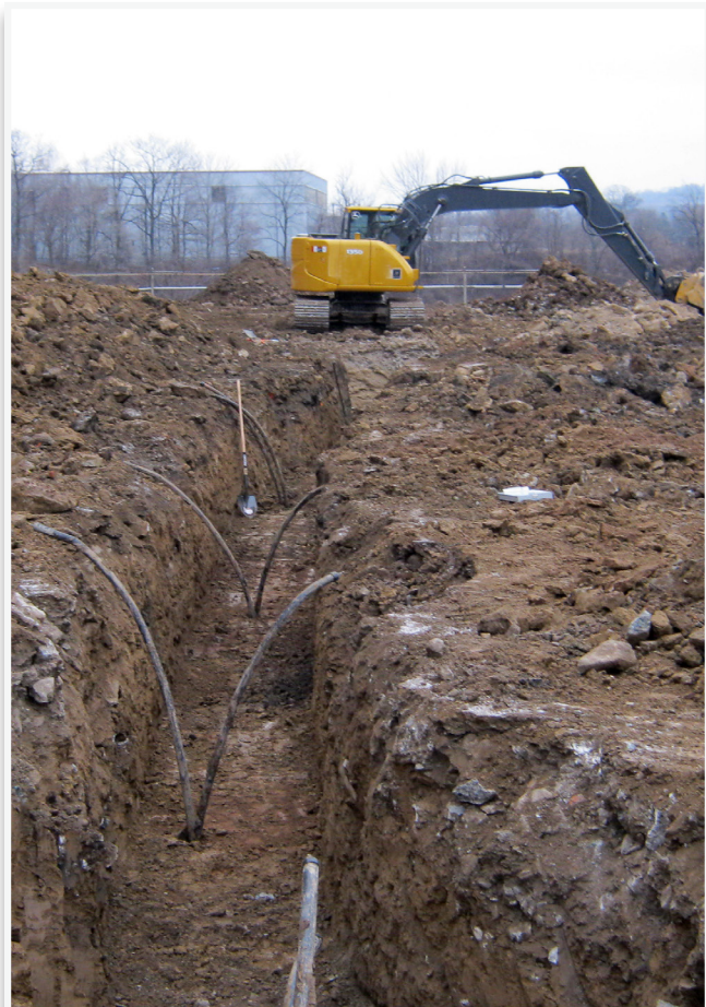
Vertical closed loop system being trenched ready for headering
