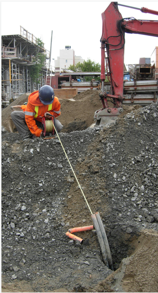
Verifying borehole depth using a dip tape
