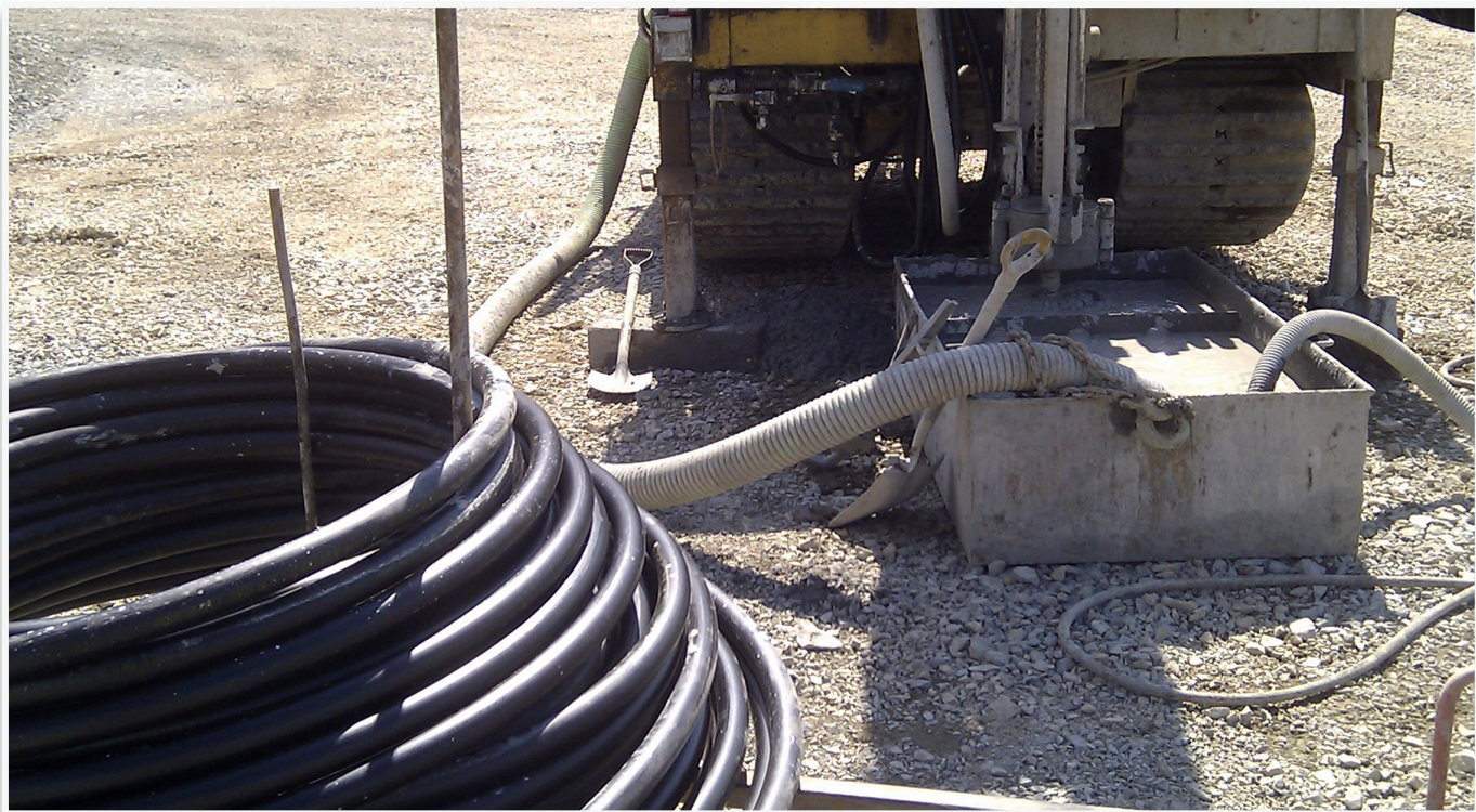
HDPE U-bend, ready to be installed
