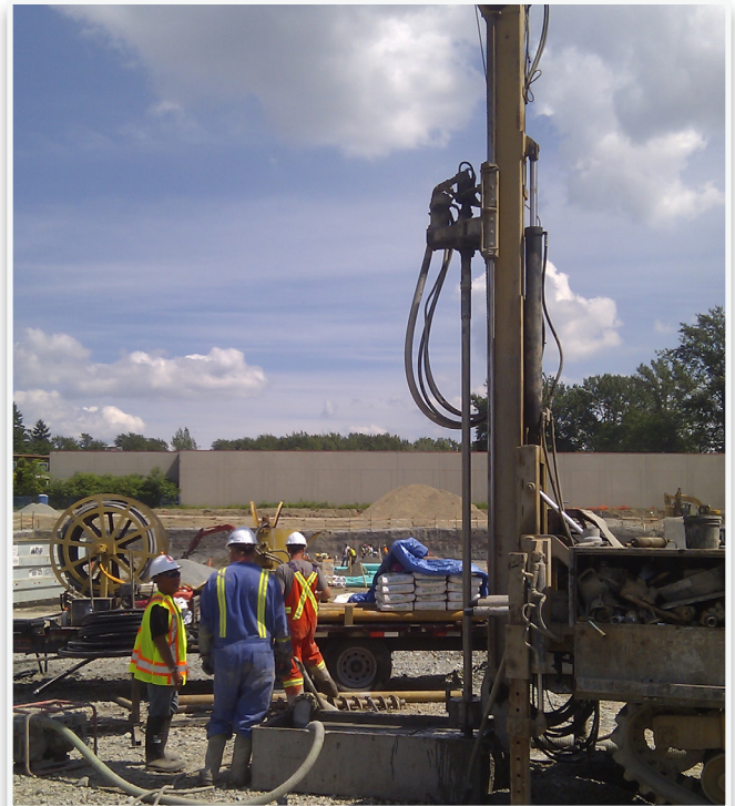
Mud rotary drill rig
