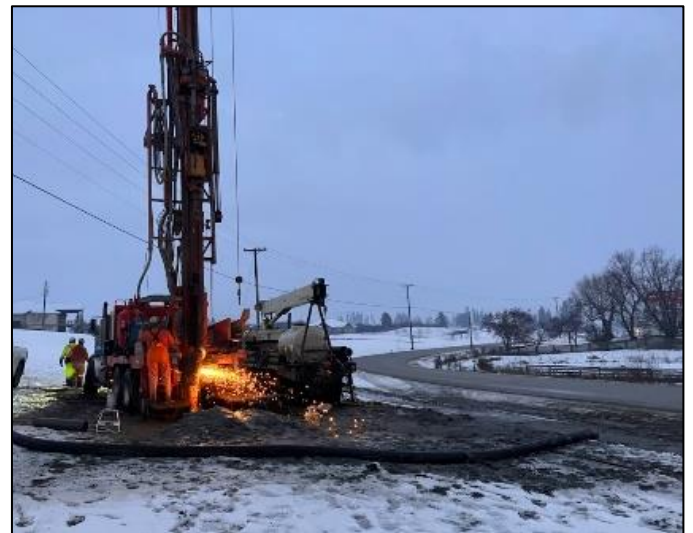
Drilling Observation Well 510 in Deep Creek (March 2023).
