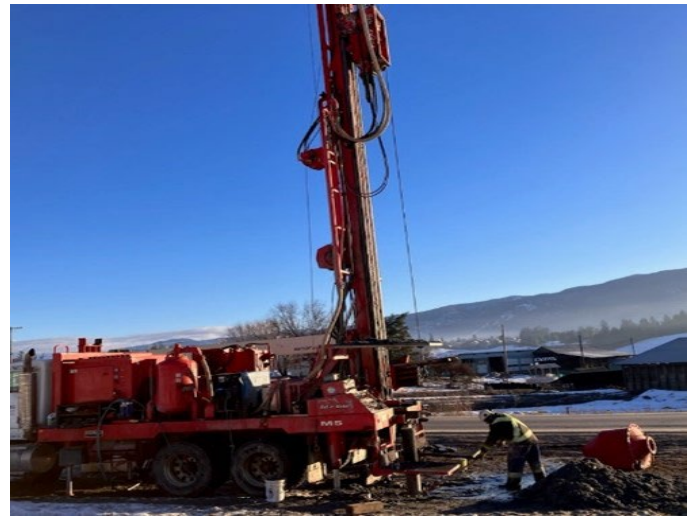
Drilling Observation Well 510 in Deep Creek (March 2023).
