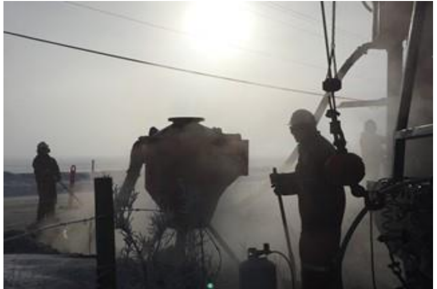
Early morning at the drill site.
